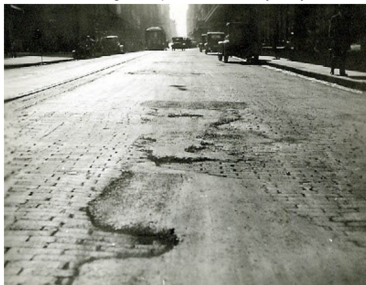
Deteriorating woodblocked road surface in Castlereagh Street, between Goulburn and Liverpool Streets, 1932. The holes have been spot filled with bitumen.
