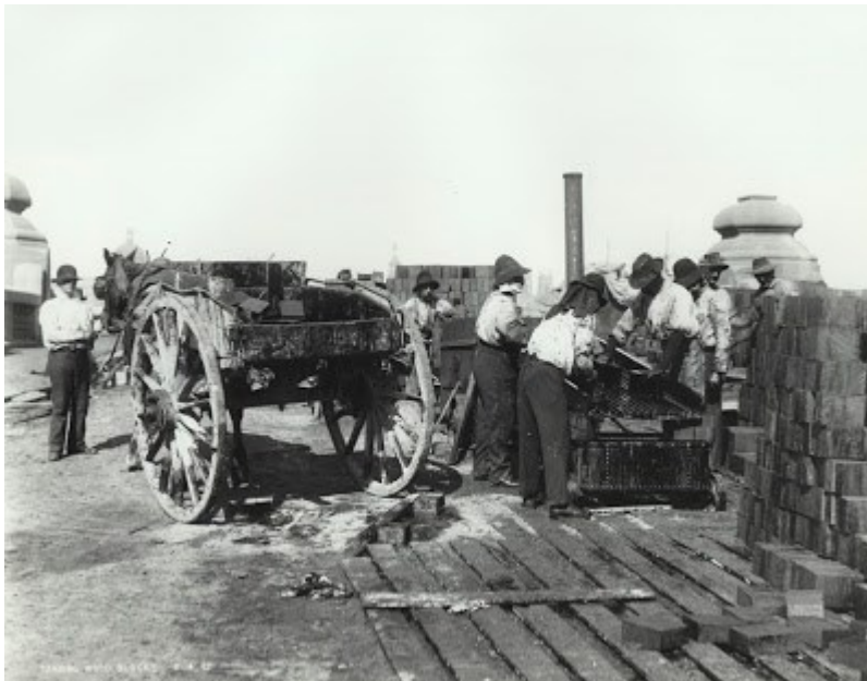
Tarring wood blocks for the construction of Pyrmont Bridge, Sydney 1902
