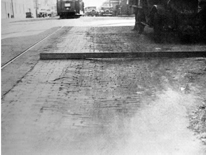
Parramatta Road, Camperdown 1931. Detail of woodpaved surface showing subsidence from heavy traffic.
