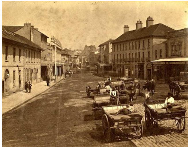
George Street, Sydney c 1880 showing stone paving prior to woodblocks
