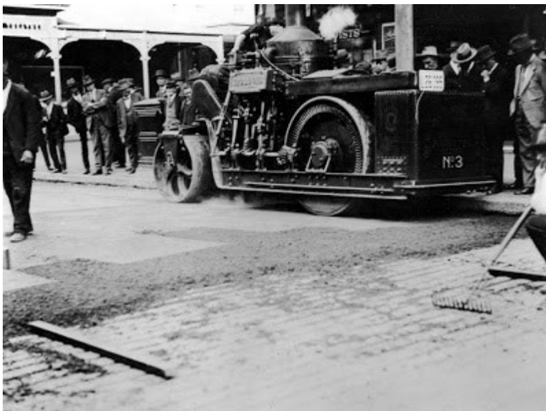
The City Engineer records the newest road-making technique being laid and tested in Park Street 1929 by the Neuchatel Asphalte Company. Woodblocked roads were gradually upgraded with asphalt from the late 1920s.
