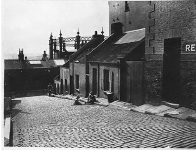
Gas Lane in Millers Point, 1909-1913, paved with woodblocks.
